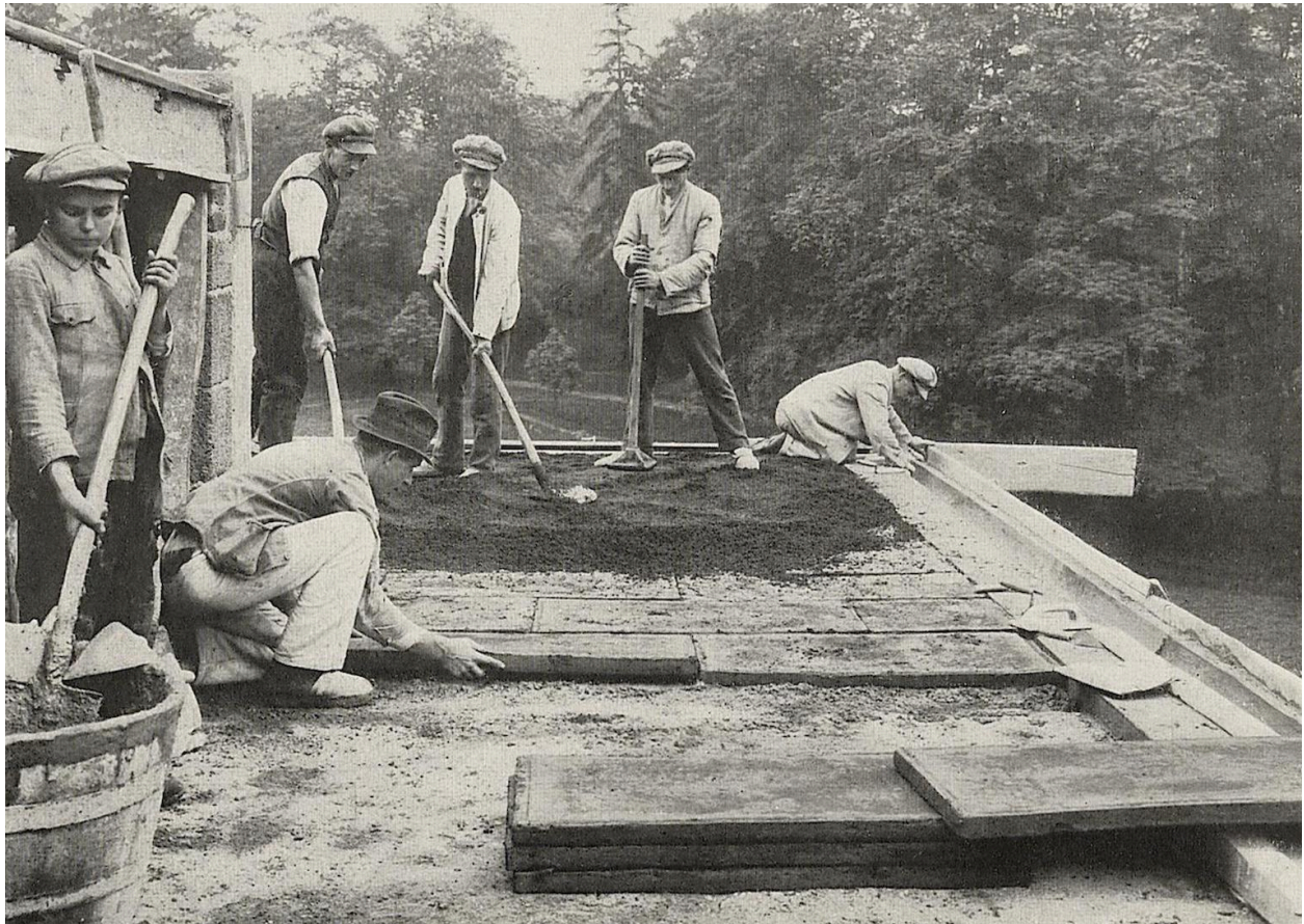
Figure 17 Figure 1 Translated caption: "Application of Torfoleum panels to the roof surfaces." Photograph from: Meyer, Adolf, Ein Versuchshaus des Bauhaus , eds. Walter Gropius and László Moholy-Nagy, Bauhausbücher 3 (München: Albert Langen Verlag, 1925), 34. Digitized by the Library of Heidelberg University.
