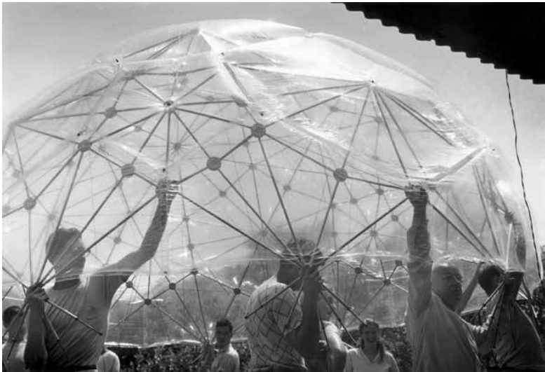
FROM LEFT: Hazel Larsen Archer, Buckminster Fuller and students constructing a geodesic dome, Summer 1949. Courtesy of the Estate of Hazel Larsen Archer.
