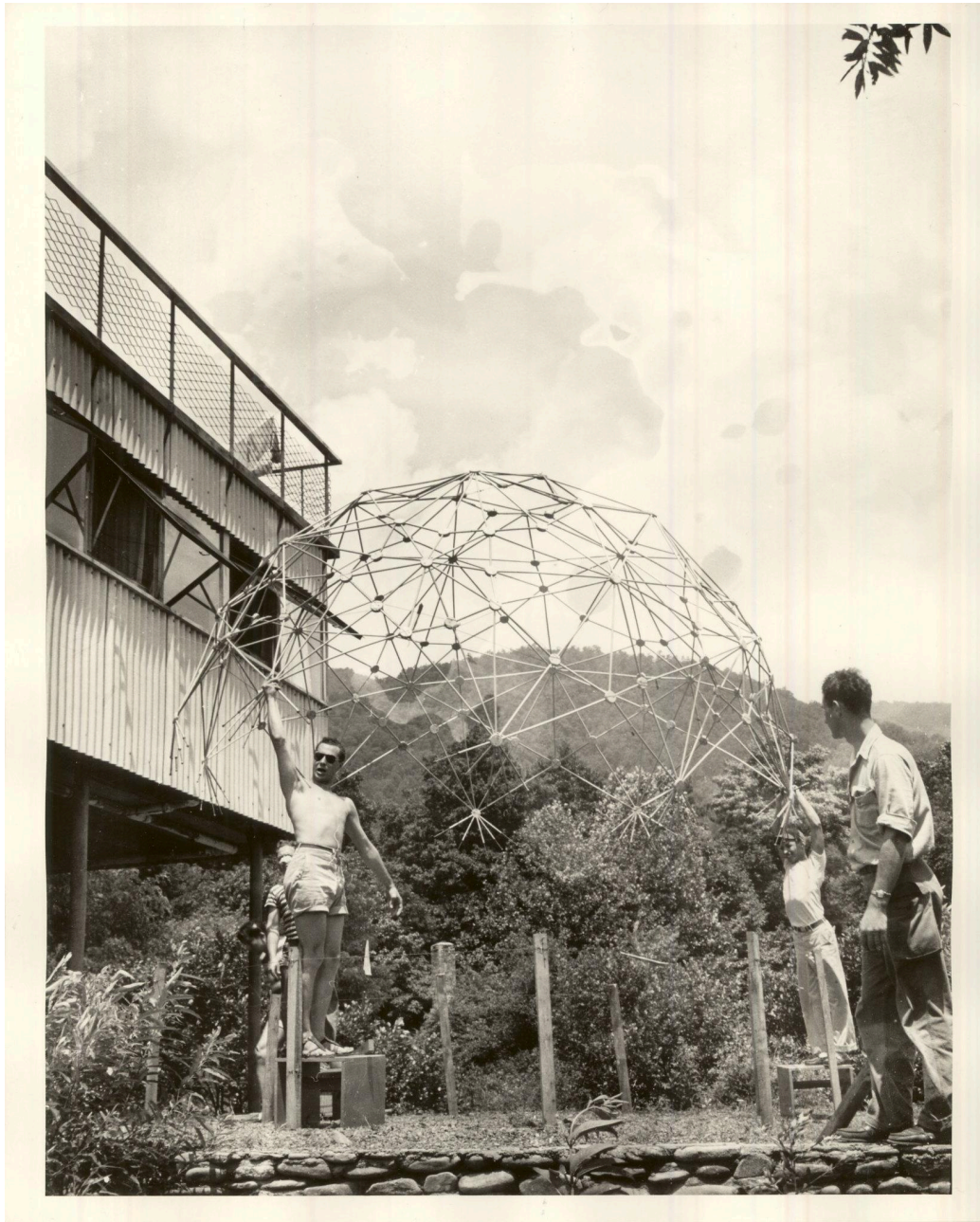
Figure 12. Students constructing the dome during the 1949 summer session. Courtesy of the State Archives of North Carolina.
