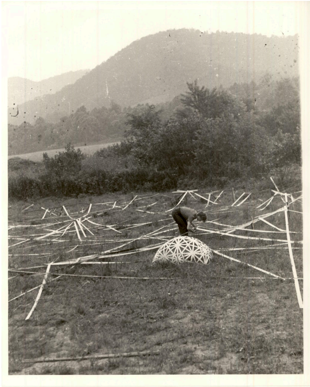
Figure 9. Venetian blind dome construction in Summer 1948, with model and Elaine de Kooning. Courtesy of the State Archives of North Carolina.
